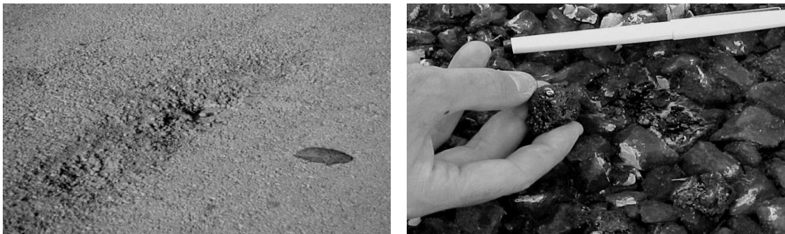
Effects of Liquid Asphalt Binder Stripping
