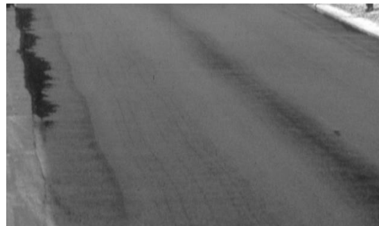
Pavement Streaking
