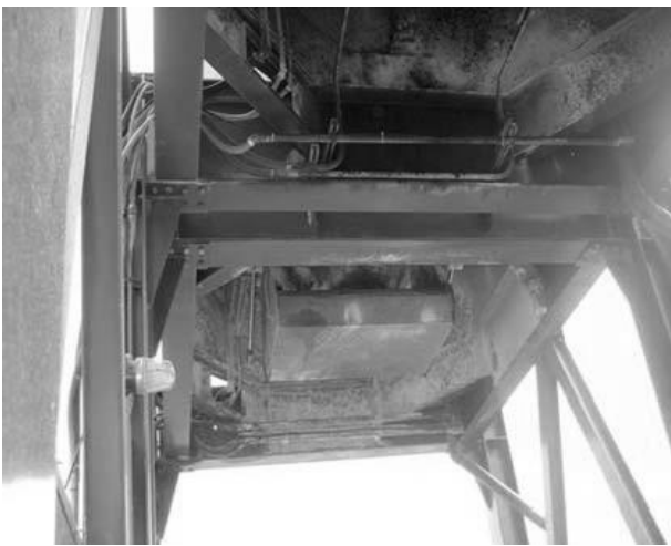
Silo Discharge Gate
