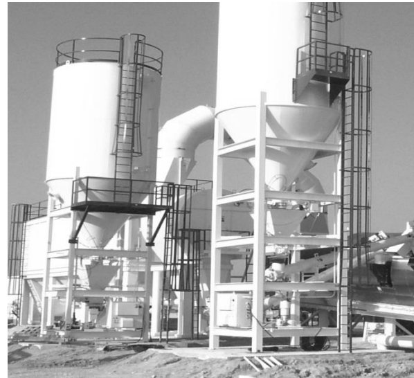
Dust storage tanks w/ weigh pod
