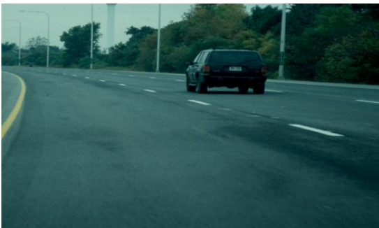
End of Load Segregation
