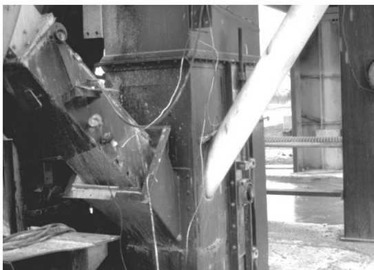
Base of the Hot Elevator
