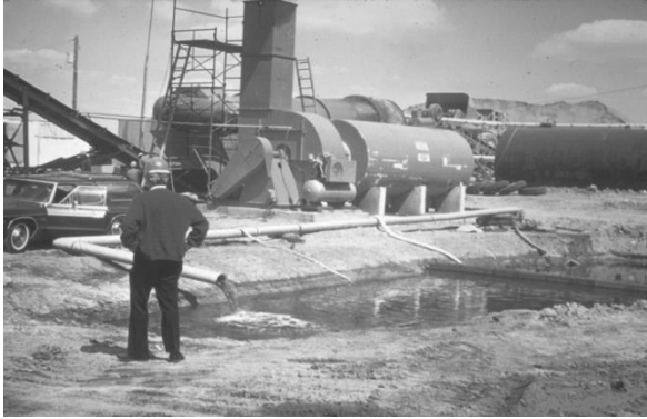
Wet-wash Dust Collectors
