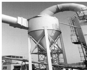
Horizontal Cyclone Collector
