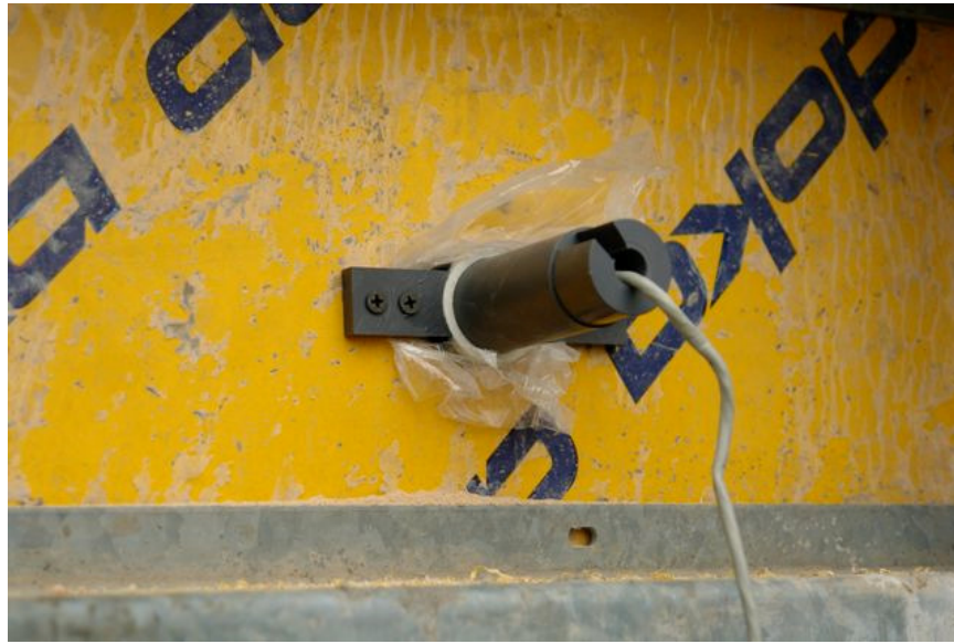
Figure 3 —Bracket with Pressure Transducer Attached to Formwork
