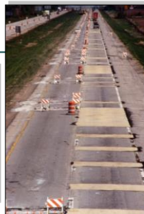
"D" Cracking
