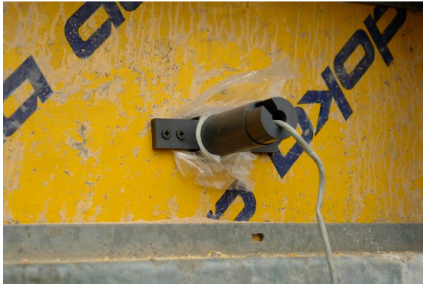
Figure 3 —Bracket with Pressure Transducer Attached to Formwork
