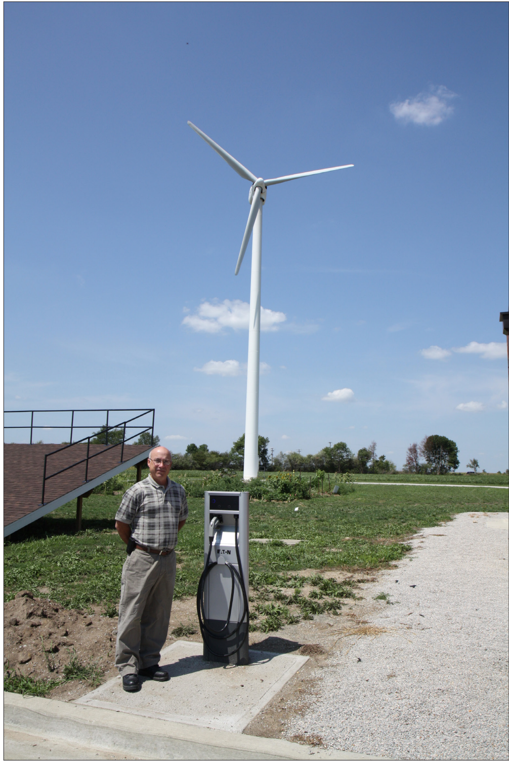
Jeff Oder, director of sustainability at Lake Land College is pictured with the college's electric vehicle charging station, which is powered by a nearby 100 kW turbine and solar panel installations.
