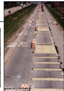
“D” Cracking
