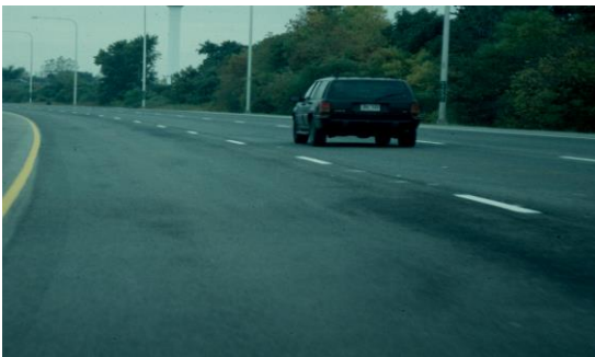
End of Load Segregation
