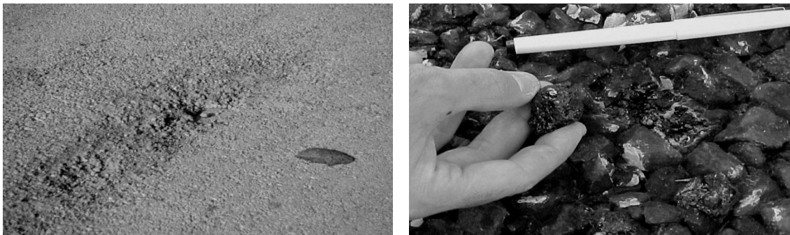
Effects of Liquid Asphalt Binder Stripping
