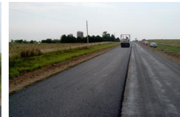
Pneumatic Roller Pass
