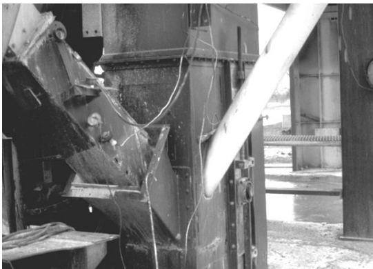
Base of the Hot Elevator
