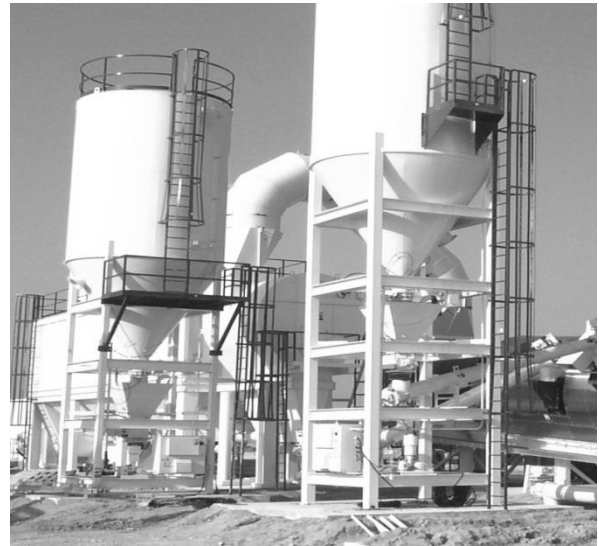
Dust storage tanks w/ weigh pod
