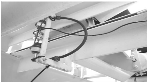
Weigh Bridge Load Cell
