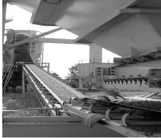
Batch Plant Cold Elevator
