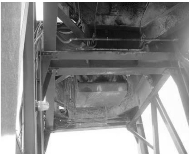
Silo Discharge Gate
