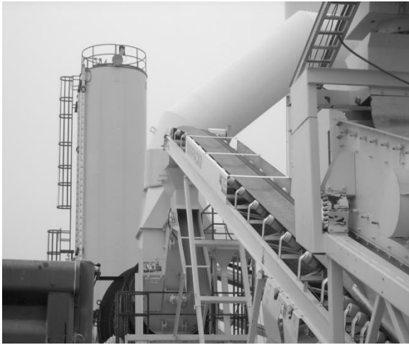
Dryer-drum Plant Cold Elevator Conveyor
